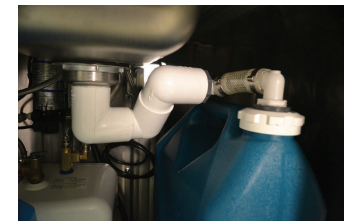
5 Gallon Container for Waste Water Shown for 26C Unit
